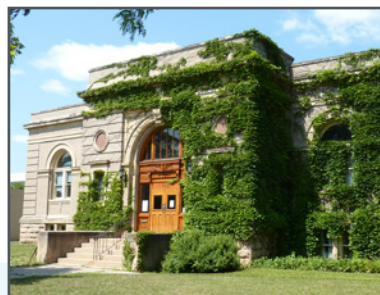
Carnegie Library in Mankato, MN
