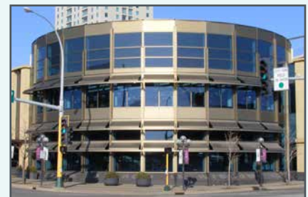
The library's fourth home opens in 1995, with initial plans for three floors, but due to budget constraints, opens with only two floors. Today the library is out of space, prompting the Library Board to move forward with plans for a 2-story expansion
